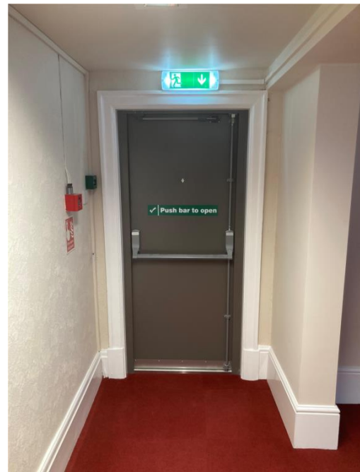
New Fire Exit Door
