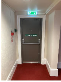
New Fire Exit Door
